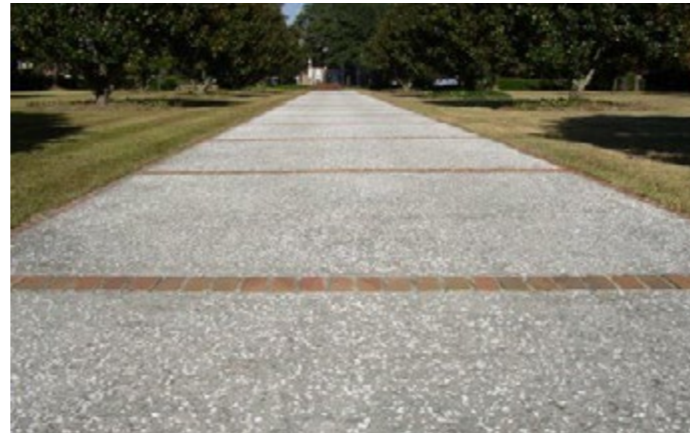
Example: Exposed aggregate concrete with feature bands to break up expanse of concrete.
