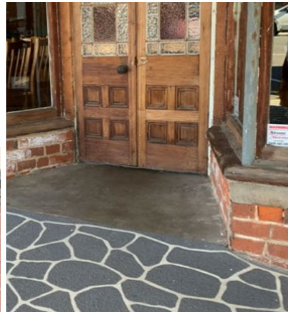
A threshold ramp seamlessly connects footpath to building entry.
