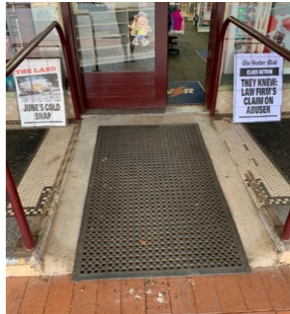
The existing ramp at the entry in Lockhart Newsagency is located within the property boundary of the shop.
