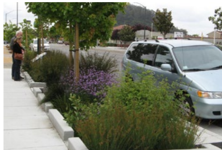
Breaks in the kerb allow stormwater to be diverted into the rain garden.
