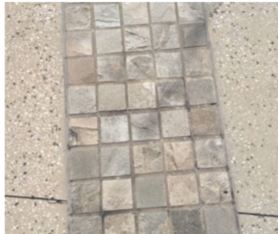
Example: Exposed aggregate concrete with feature bands to break up expanse of concrete.
