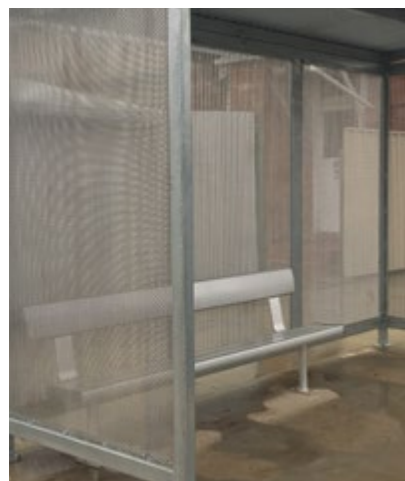
Galvanised steel with perforated screens is a simple and contemporary design which works well in the heritage setting.
