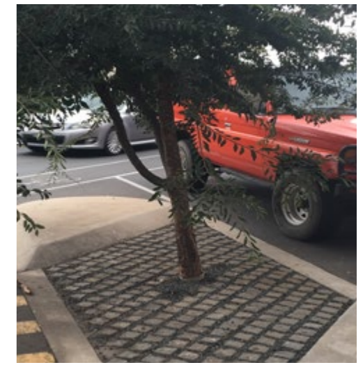
Street trees in permeable paving (such as granite sets or bonded gravel). Raised concrete section close to the road protects the tree from vehicles.
