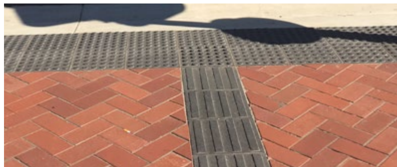
Hazard dot and directional tactile pavers assist access for vision impaired.
