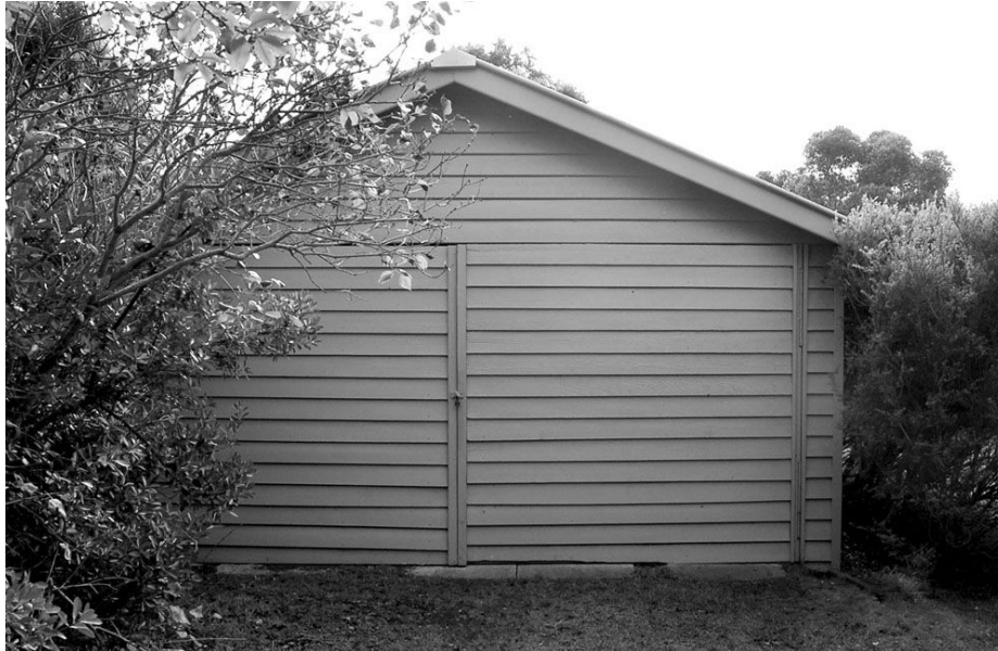
Door in weatherboard wall
