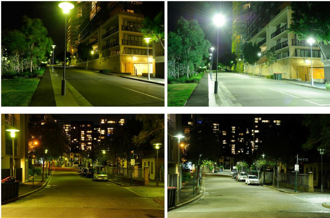
ABOVE: PHOTOS OF SUBURBAN STREETS IN SYDNEY BEFORE AND AFTER THE AFTER THE TRANSITION TO LED LIGHTING. THE LED LIGHTING IS FAR MORE EFFECTIVE WITH FAR LESS UPWARD LOSS OF LIGHT.
