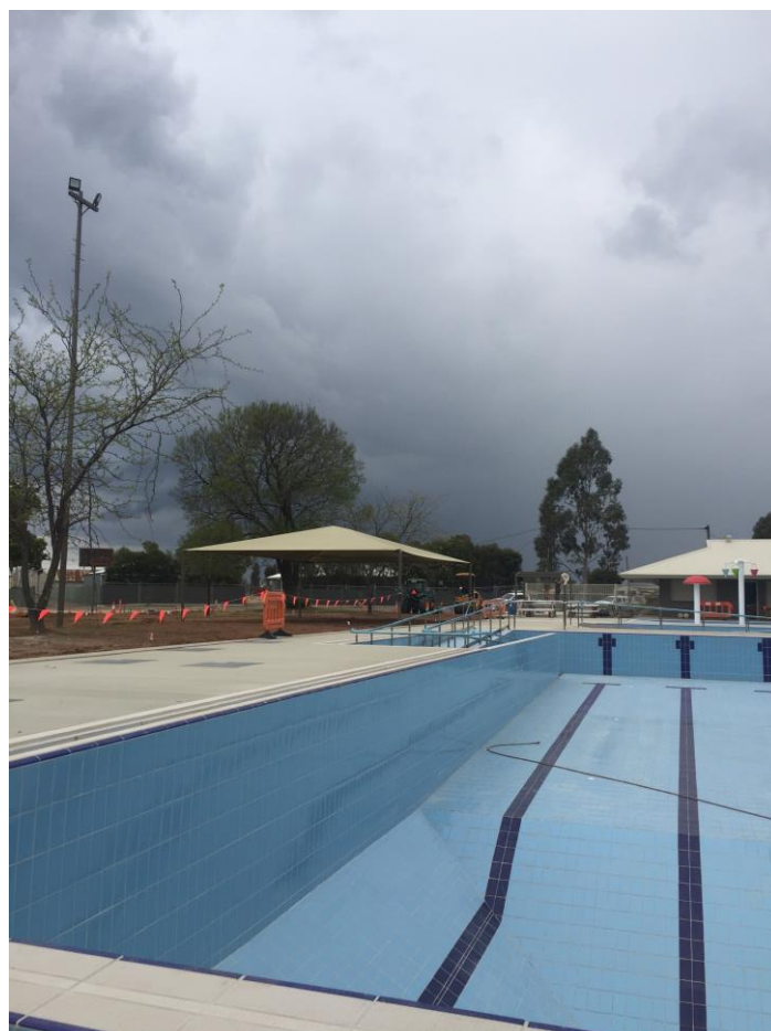
New Lockhart Swimming Pool with all abilities access under construction
