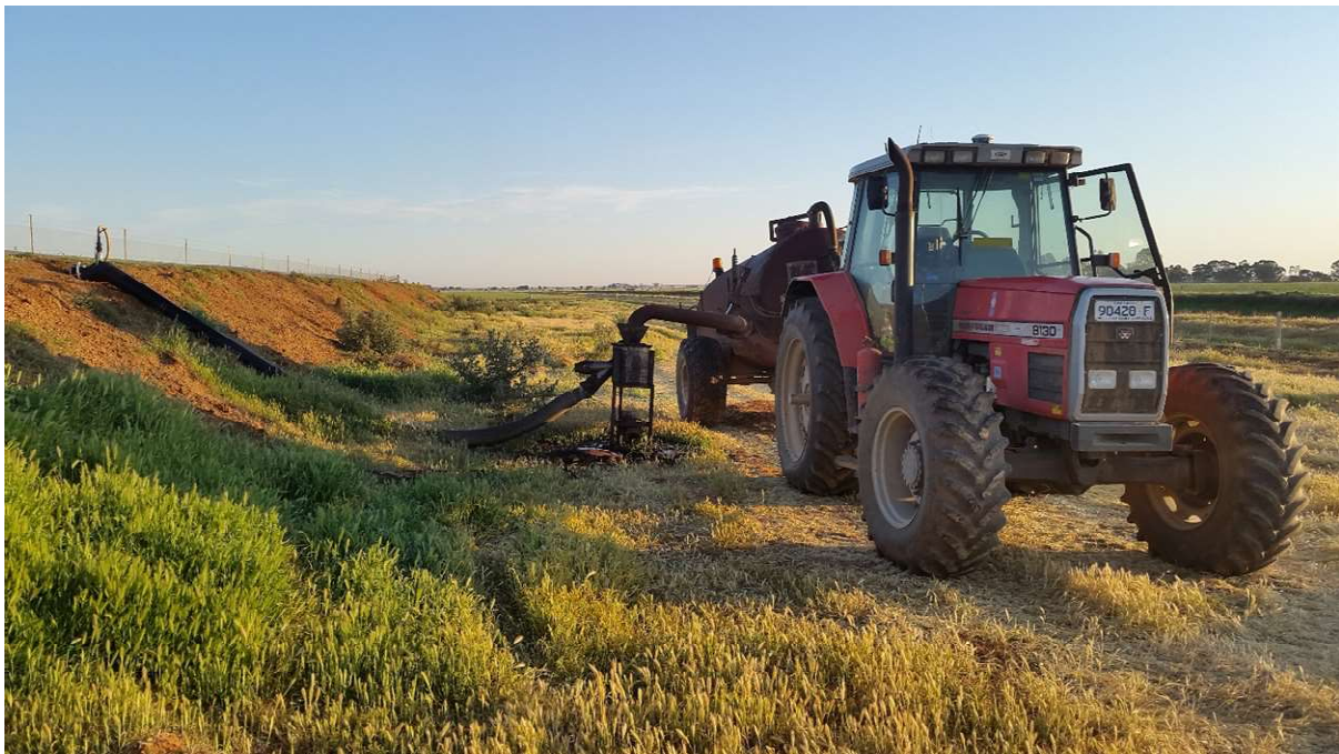
Photograph 4 – Pond Desludging Infrastructure
