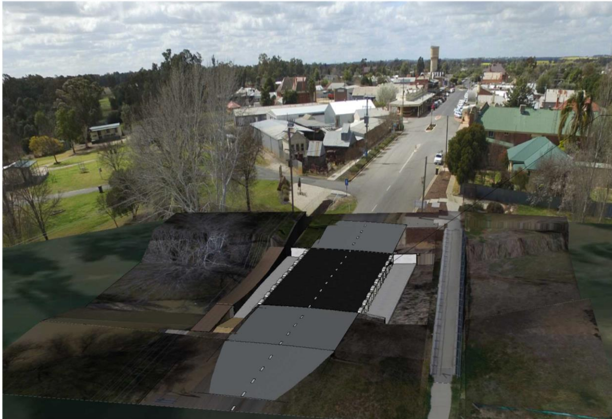
Proposed 19.8 long by 12m raised 600mm new culvert crossing at Green Street Lockhart
