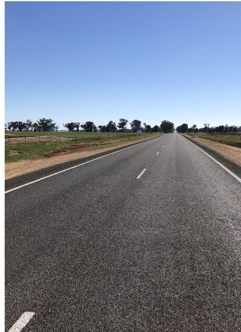
Rehabilitation of a section of Albury Road was completed in February 2022.
