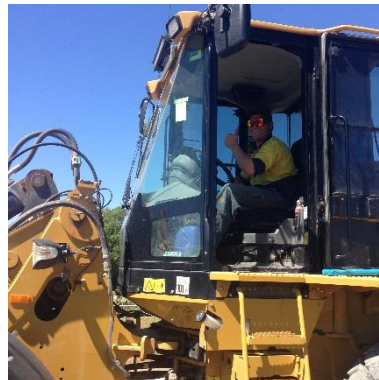
Lockhart Shire Council Road Crew on the job
