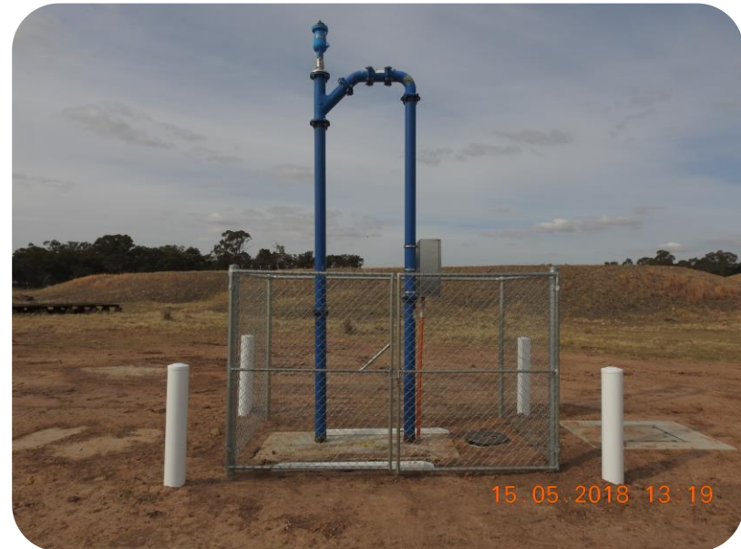
Barametric Loop – The Rock East Sewer Scheme
