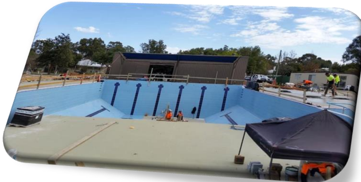
Refurbishment works, Lockhart Swimming Pool Complex, officially opened 27 October 2018
