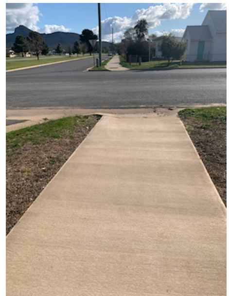
New Footpath Construction, Urana Street, The Rock
