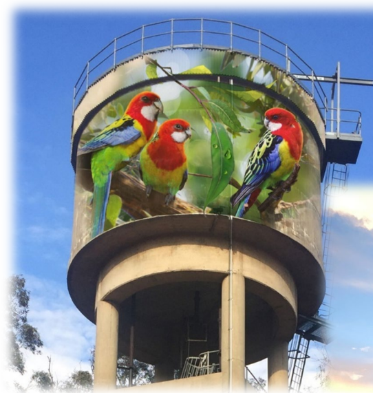
Milbrulong Water Tower
