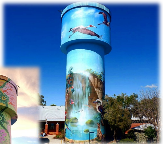
Lockhart Water Tower
