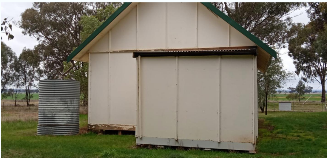
Figure 7: The view east from the rear of the Church.
