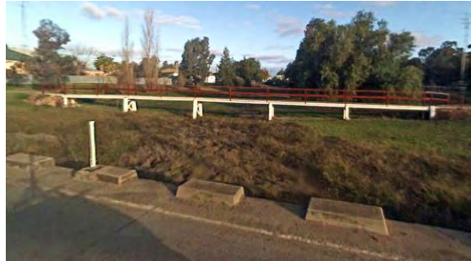
Image 10: Green Street Footbridge pre March 2012 Flood (source: Google Earth)
