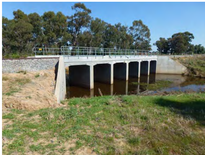
Image 12: Oaklands Railway Bridge (source: Reference 3)
