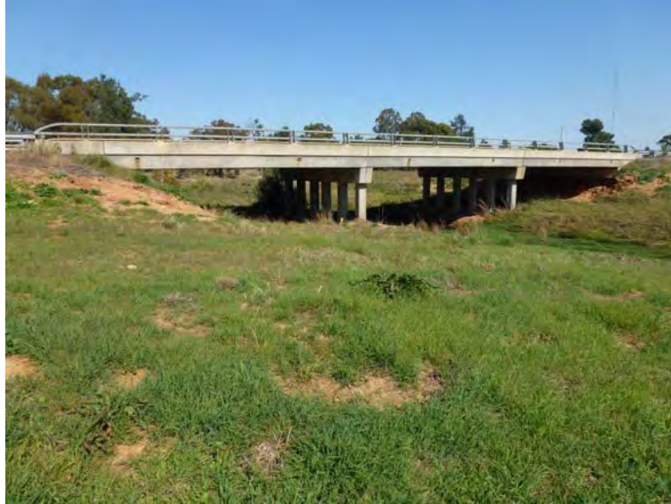
Image 13: Urana Road Bridge (source: Reference 3)
