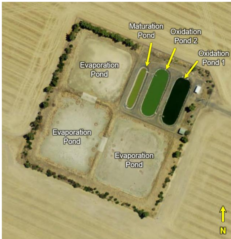
Figure 4-10: Aerial photograph showing layout of Yerong Creek STP
