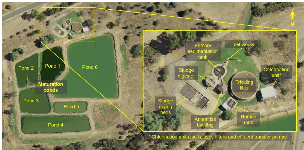
Figure 4-3: Aerial photograph showing layout of Lockhart STP
